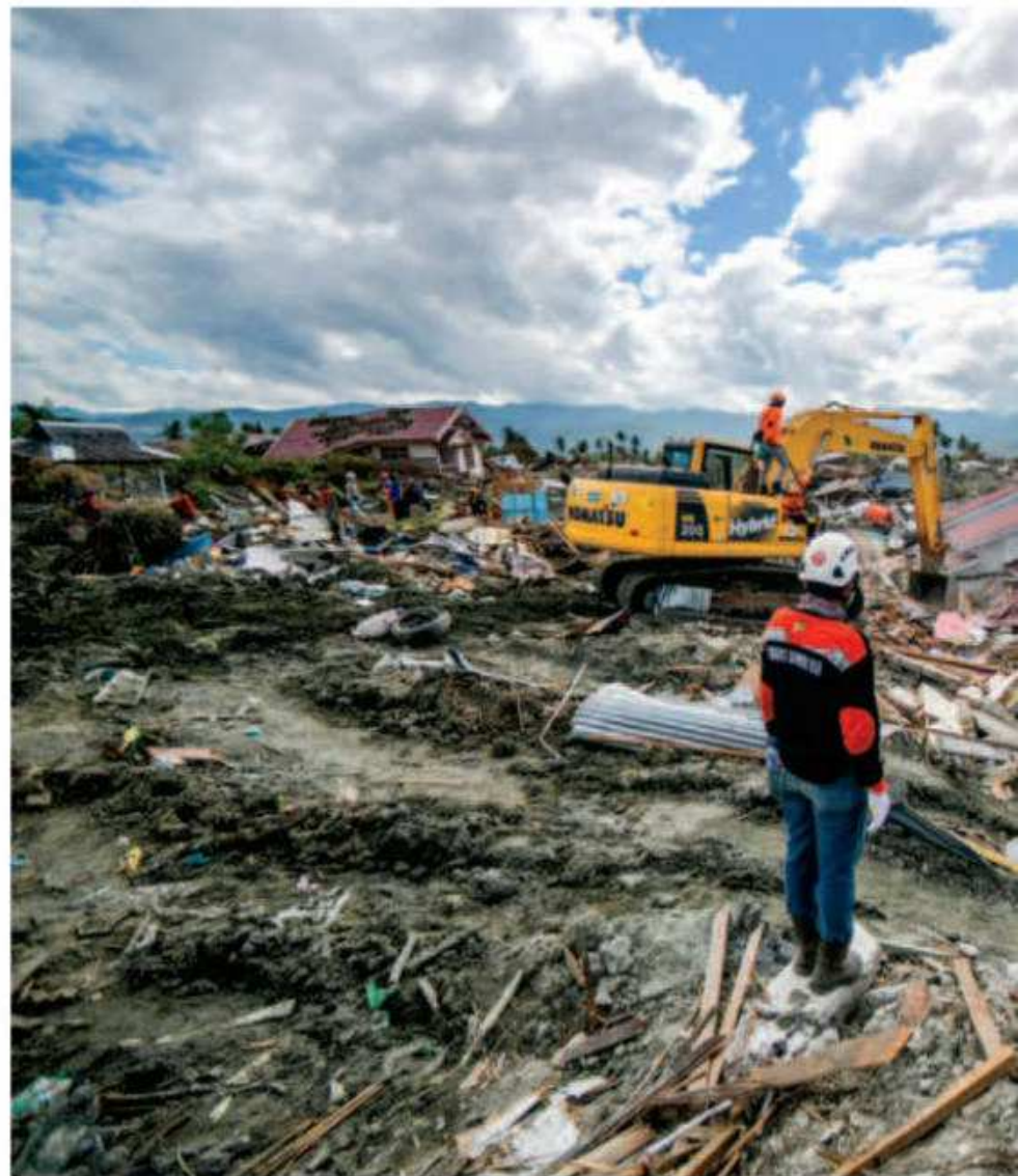
▲ A search-and-rescue team works to recover bodies from the debris in Petobo on Oct. 8
